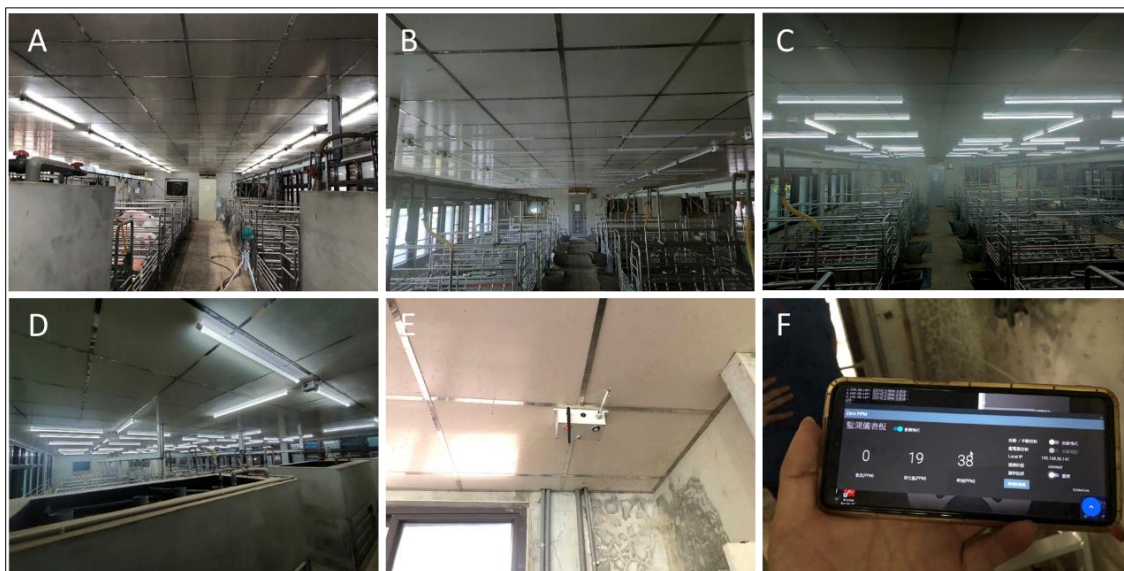
Figure 1 Progression of installing and employing the state-of-the-art LED lighting system and harmful substance sensors within a specific pathogen-free pig farm. (A) Before Installation of LED lighting system in the animal housing facility. (B-E) After Installation of LED lighting system and integration of harmful substance sensors in the animal housing facility. (F) Testing conducted subsequent to harmful substance sensor installation in the animal housing facility
