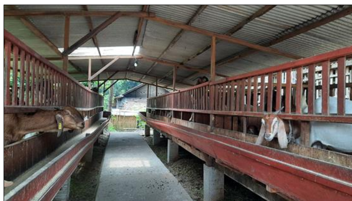
Figure 3 The condition of goats rearing cages in Sun Farm
